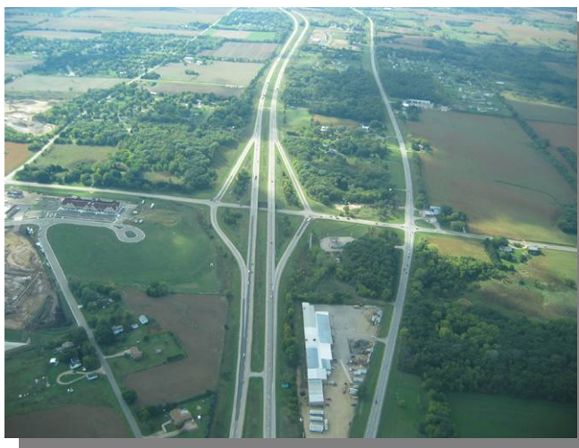
Looking west along Interstate 94
