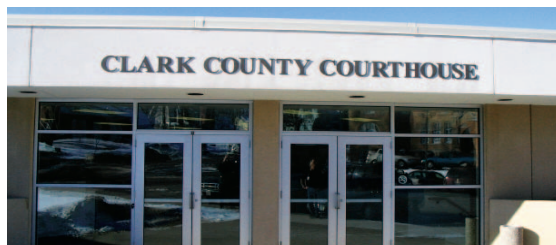
The Clark County Courthouse project involved replacing T12 fixtures with T8 energy efficiency options.
